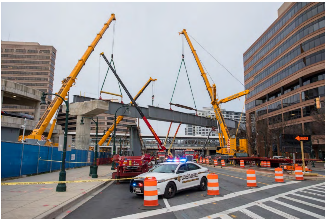
Figure 2.3-19: Elevated Guideway Construction
