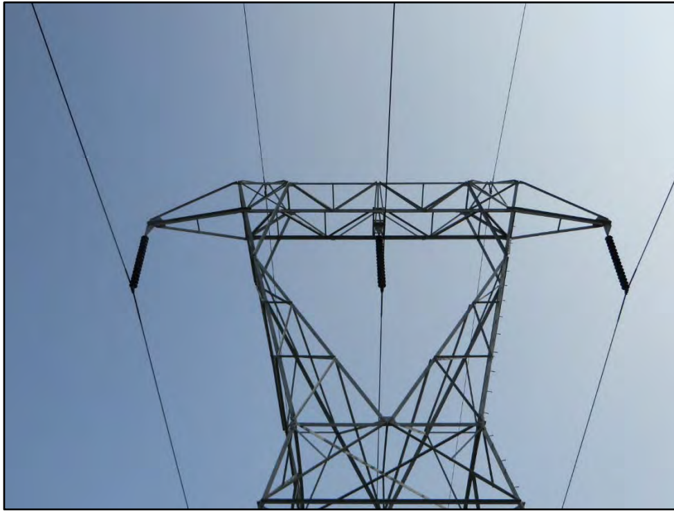
Photograph 13. Upward detail view to northeast of upper part of north tower in 3/5 pair, showing typical arrangement of three conductors with vertical insulator strings, and two grounding wires at top.
