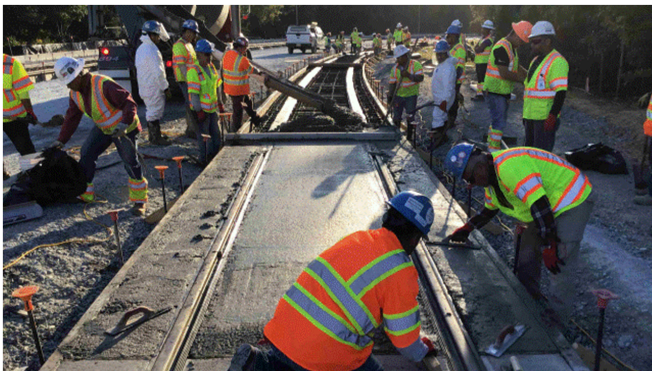
Photo 2: Placement of embedded track in Ellin Road near Veterans Highway
