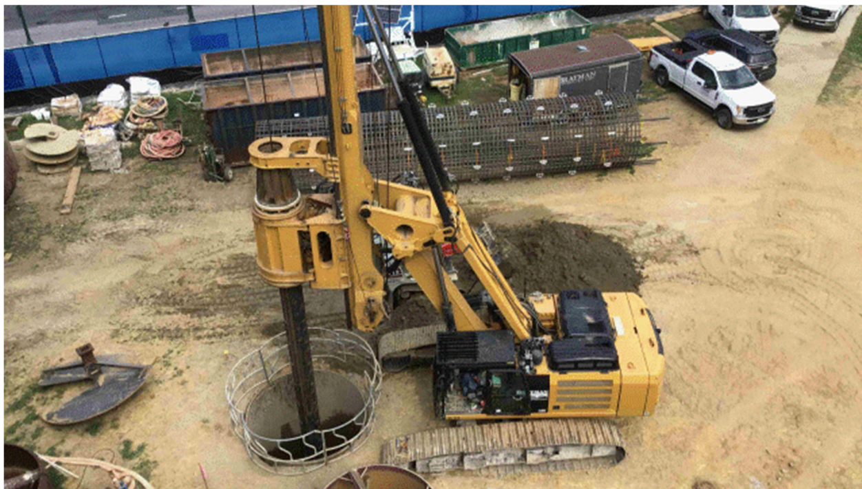
Photo 1: Drilling shafts for piers of the LRT aerial structure at the Silver Spring Transit Center
