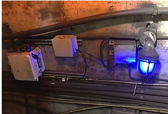
Figure 3-6 Wayside unit installed in WMATA tunnel environment
