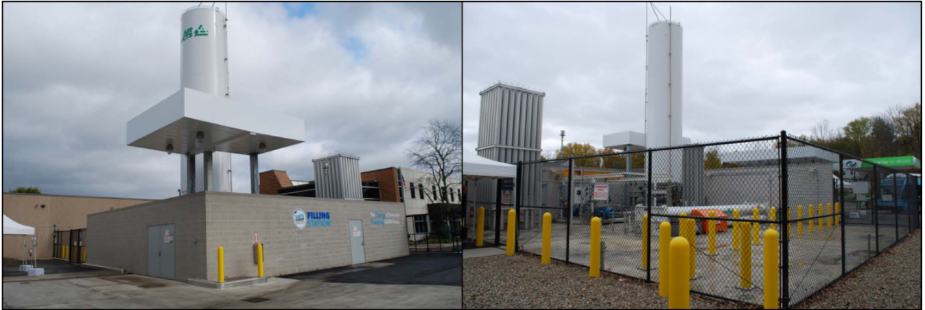
Figure 2-4 SARTA Hydrogen Station
